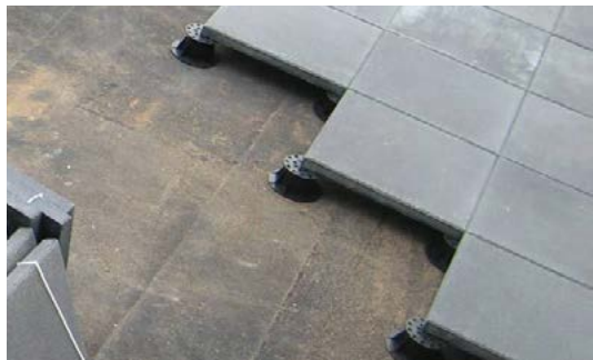
PEDESTAL PAVING, CONCRETE PAVERS
